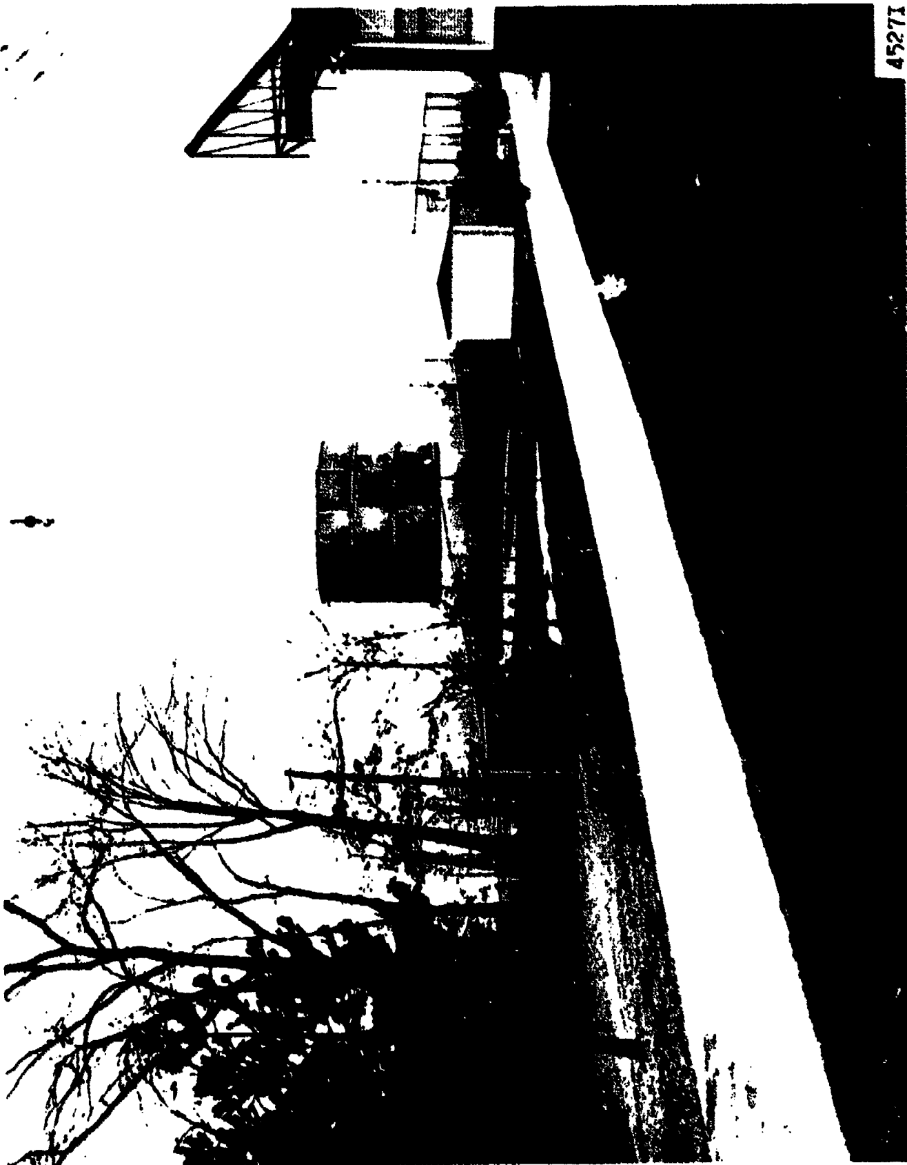
Storage Tank Being Lowered Onto Its Pad by Crane
