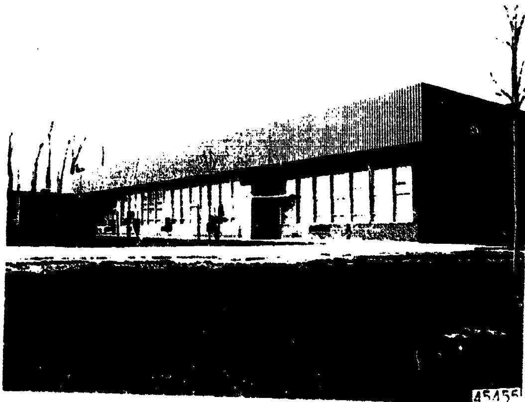
Wing of School After Solar Heating Installation Showing Screen
