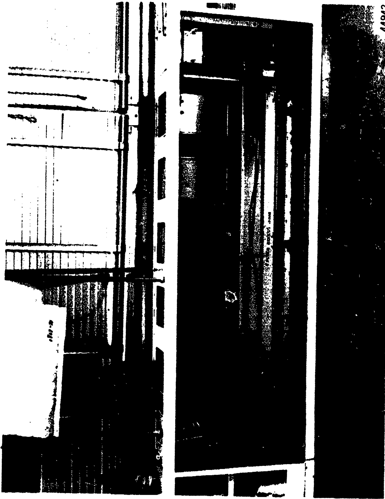
Heating and Ventilating Steam Unit With Protective Cover Removed
