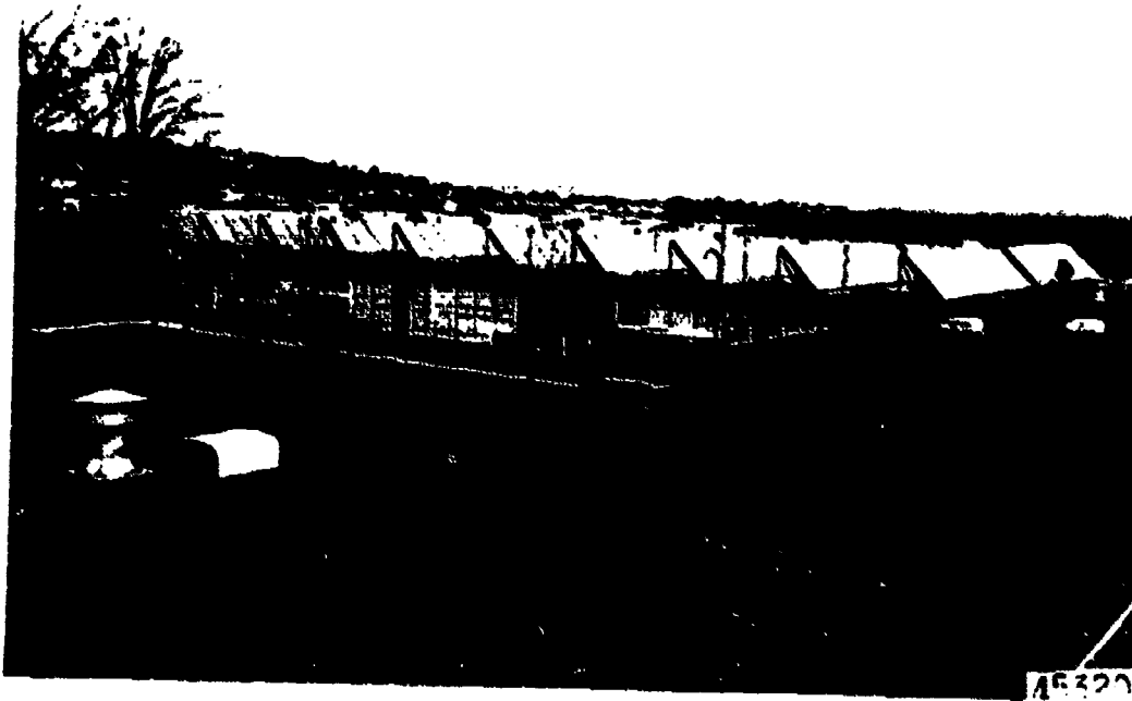
Solar Array of 180 Collectors
